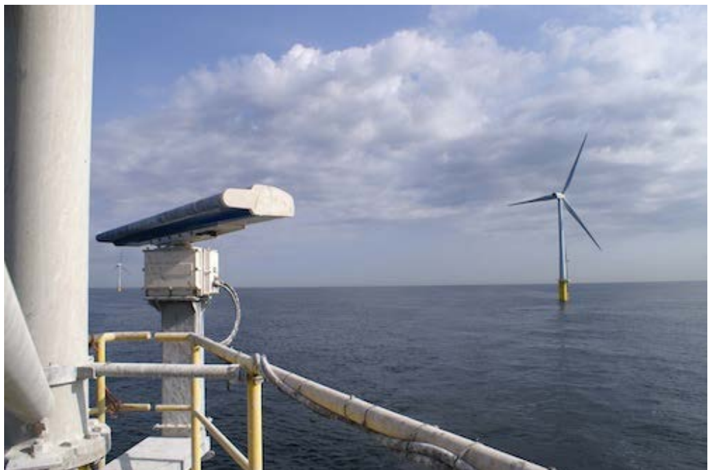
Horizontal radar on the metmast (photo Ruben Fijn)
