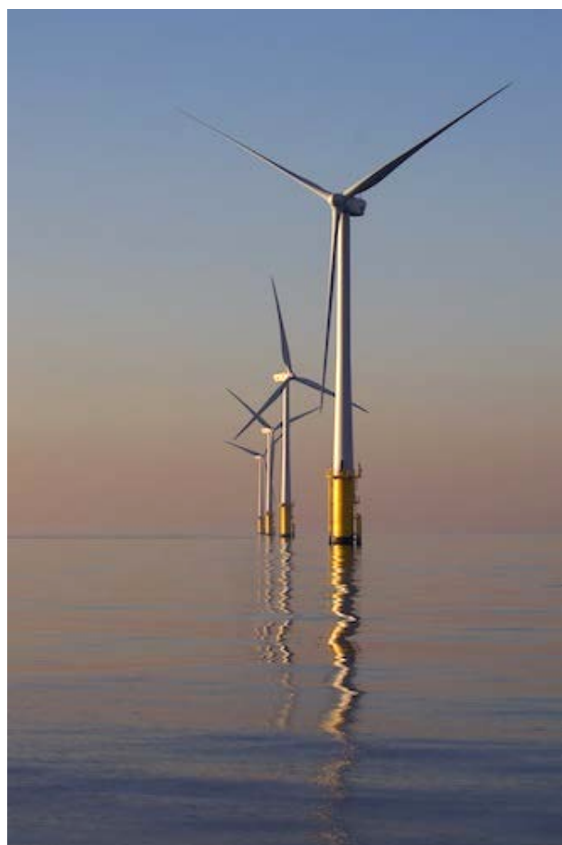
Row of turbines in the OWEZ wind farm (photo R. Fijn)
